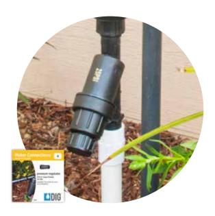
Pressure regulators are a key component to any drip irrigation system. Their function is to reduce and regulate the incoming water pressure entering a drip irrigation system to the recommended operating pressure of 25 PSI. Using a pressure regulator will help to ensure that all components operate correctly.
